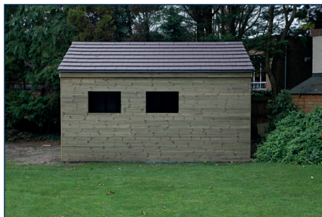
Fig. 7: October 23 rd . At least the lab now has a fine roof, even though it is still waiting for windows and doors.
