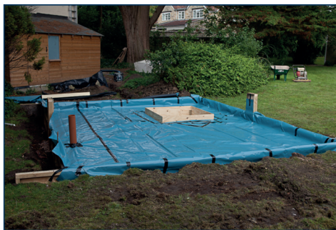
Fig. 6: September 8 th - Damp proof membrane covering the insulation for the raft, prior to pouring the concrete. Note the drain pipe on the left, and the shuttering for the extra-deep pedestal under the column.
