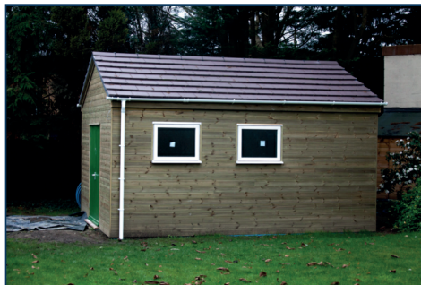
Fig. 8: December 13 th . The lab now has doors and windows, and the dry lining is nearly complete. Also, much of the electrical cabling has been run.
